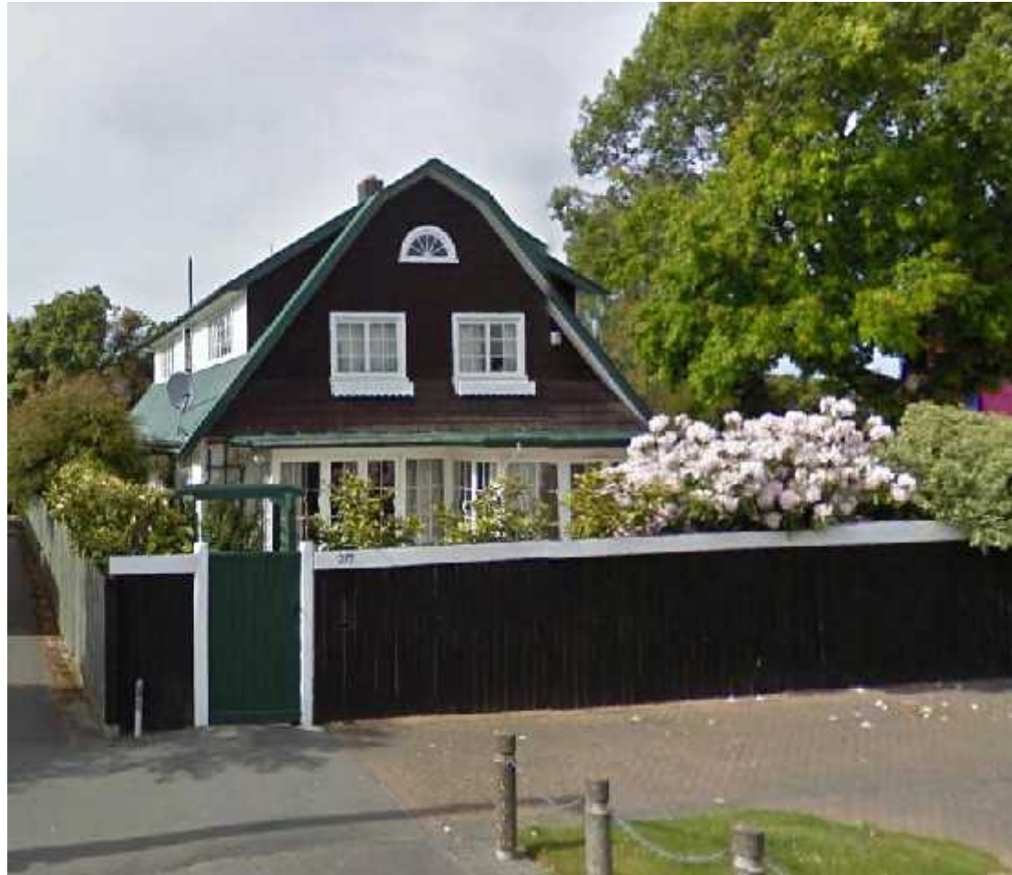
Dr King's house in Rangiora, built ca. 1928
